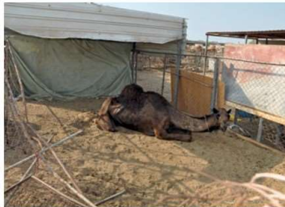
Figure 12: Broken fence: Partly collapsed fencing risking injury. The camels may escape.
